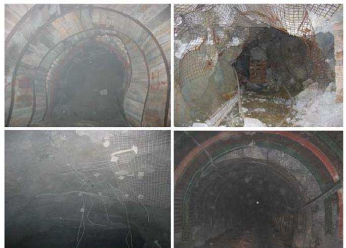
Figure 1. Drifts with stability problems of different types such as collapses and high deformation.
