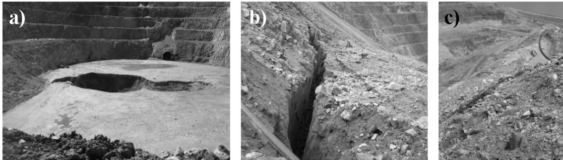
**Figure 7** Early affections of subsidence in Tinyag: a) Chimney caving in the floor of the Tinyag pit a few weeks after underground mining SLC started, b) Tensile opening of bedding planes in quartzite due to toppling in the east slope and c) detail of toppling in the east open pit wall.
