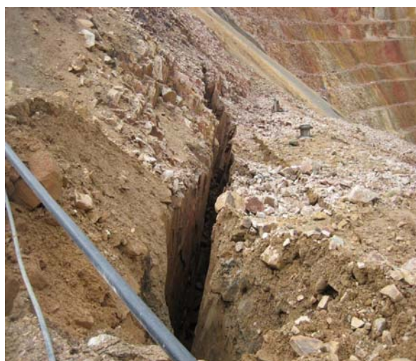
Figura 15. Tensile crack in a slope of the Tinyag mine.
